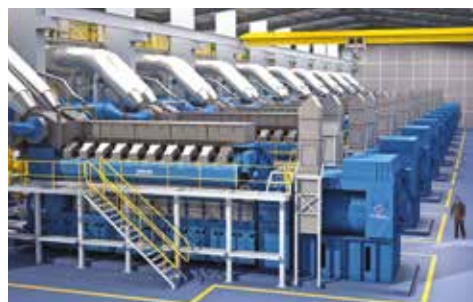
"The Power of 10". A modular Microgrid power solution incorporating 10MW Bergen engines, Marelli generators & Piller power conditioning technology for rapid deployment of power at scale.
