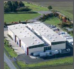
Piller Assembly & Testing Facility, Bilshausen, Germany
